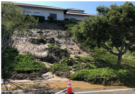
Surficial Slope Failure Caused by Heavy Rain
