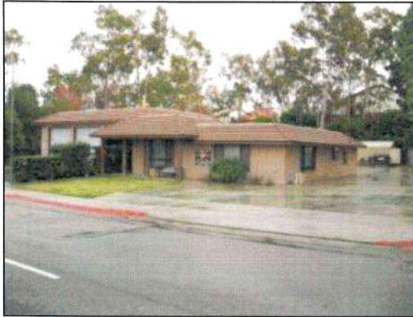
Photo 13 – Fire Station #4 A general view of the front entrance of the fire station.
