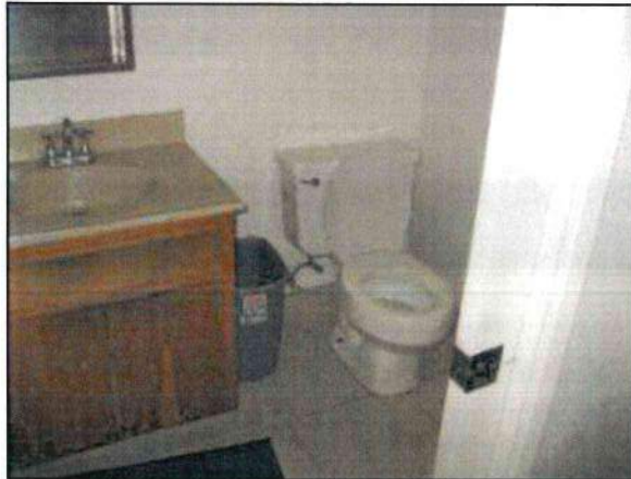
Photo 69– Fire Station #4 A general view of the restroom off the game room.
