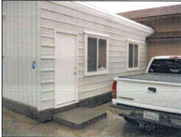
Photo 37– Fire Station #4 A general view of the steel metal addition attached to the rear of the building.
