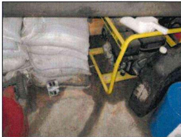
Photo 52 – Fire Station #4 Major leaks are present on the inside rear of the shed.
