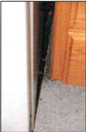
Photo 47 – Fire Station #1 Heavy debris has accumulated beside the refrigerator. The debris may attract pests.
