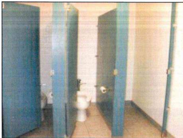
Photo 27 – Fire Station #1 A general view of the commodes in the locker room and general conditions.
