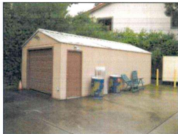
Photo 48 – Fire Station #4 The storage shed located at the rear of yard is sheathed in T-111 masonite and has a steel roof, steel entry door, and an aluminum roll-up door.
