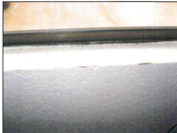
Photo 60 – Fire Station #4 The windows in the bedrooms are fitted with drywall window sills. The drywall is drag stucco and paint.
