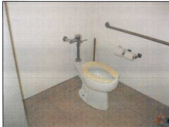
Photo 70 – Fire Station #4 A general view of the main restroom and commode.
