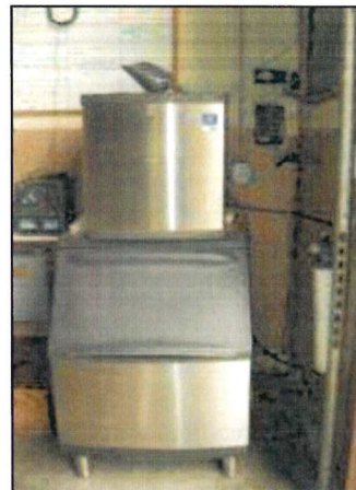
Photo 8 – Fire Station #4 An icemaker is present in the garage. The unit required cleaning at the time of the inspection.
