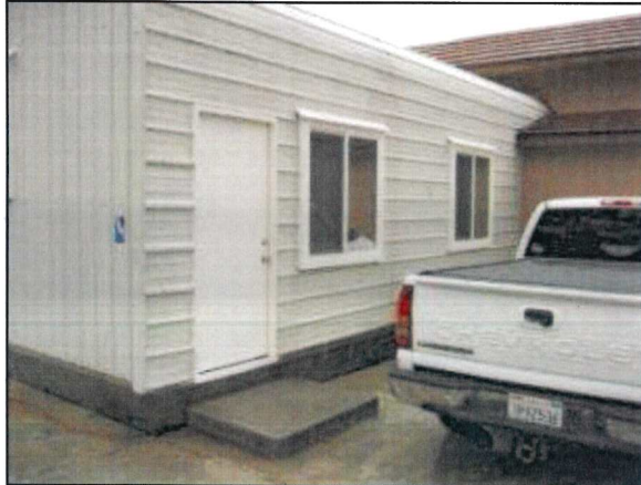
Photo 37– Fire Station #4 A general view of the steel metal addition attached to the rear of the building.
