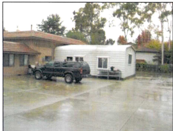
Photo 16 – Fire Station #4 A general view of the rear of the building showing the later addition.
