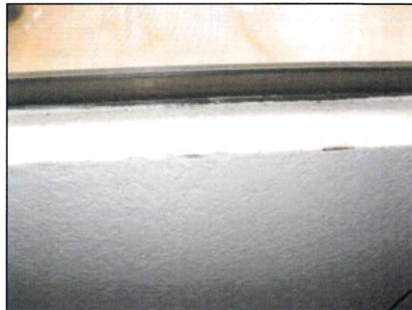
Photo 60 – Fire Station #4 The windows in the bedrooms are fitted with drywall window sills. The drywall is drag stucco and paint.
