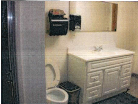
Photo 25 – Fire Station #1 A general view of the captain’s restroom and general conditions.
