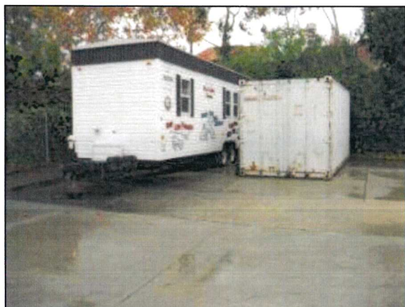
Photo 53 – Fire Station #4 A trailer and storage shed are present at the rear corner of the fire station lot.
