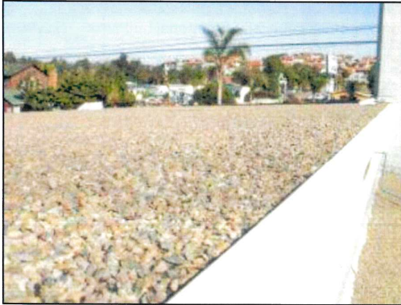
Photo 1 – Fire Station #1 The fire station exhibits a flat structure built up roof with gravel aggregate.
