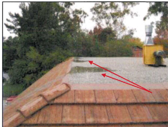
Photo 20 - Fire Station #4 Standing water was noted on the flat portion of the roof at the time of the inspection.
