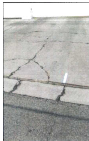
Photo 28 – Fire Station #1 The concrete at the garage is severely cracked and deteriorated. Loss of underlying support is also evident.
