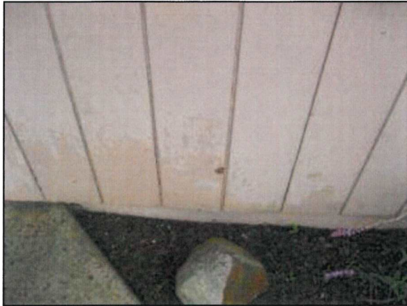
Photo 33 – Fire Station #4 The fire station structure is sheathed in 5/8" T-111 plywood siding.
