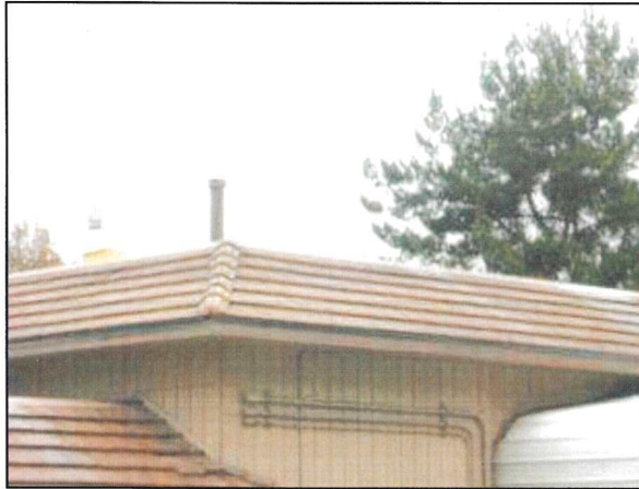
Photo 5 – Fire Station #4 The garage is ventilated by means of a vehicle exhaust system that is mounted on the roof. The system is similar to that present in Fire Station #5.
