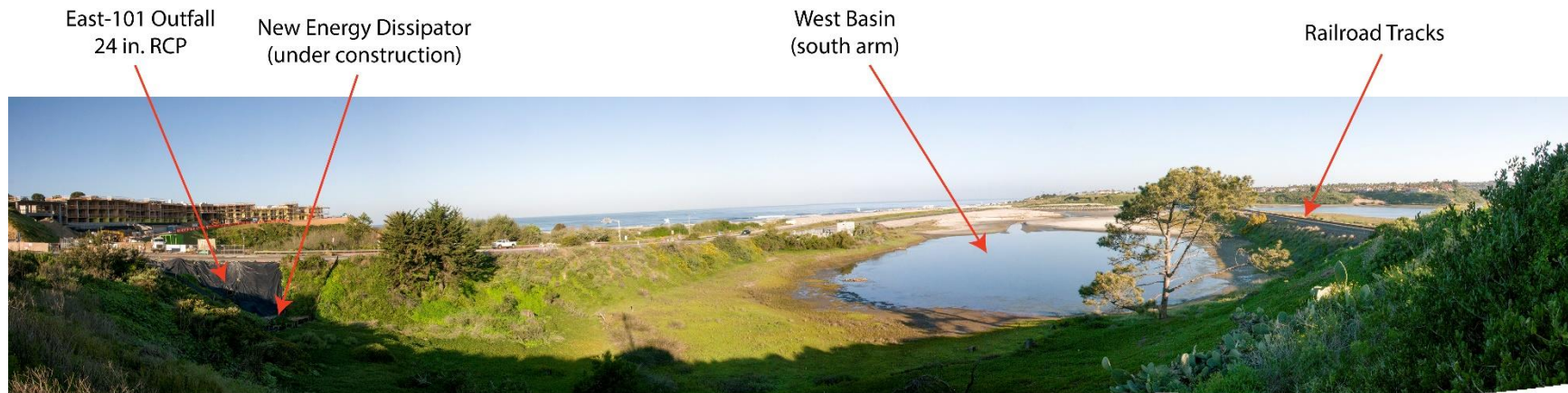
Figure 1: View of major components of the North Coast Highway 101 infrastructure improvements in the south arm of the West Basin of Batiquitos Lagoon including East 101 Outfall enhanced by new energy dissipator,
