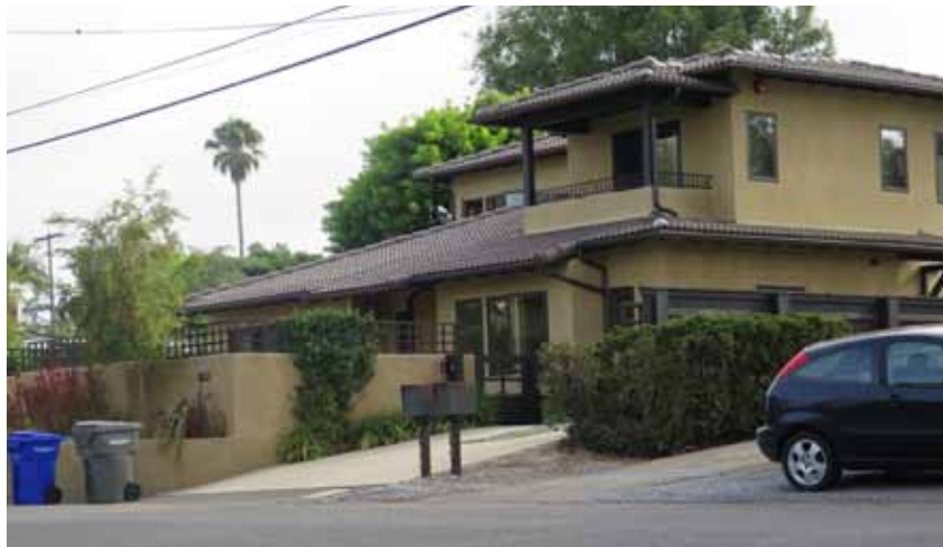
Terrace development on steep slopes, following the natural contours of the site.
