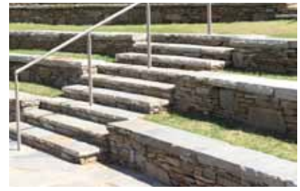
Terrace a retaining wall on a steep slope to minimize the height of individual walls.
