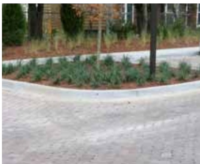
Use permeable materials for portions of a surface parking lot in order to reduce on-site run-off.
