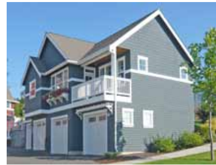
Carriage houses provide parking for larger residential prototypes while providing a sensitive transition to single family.
