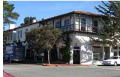
New building materials should contribute to the visual continuity of the community character.
