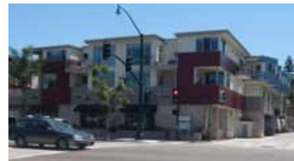
Vary the roof profile by stepping down some parts of the façade
