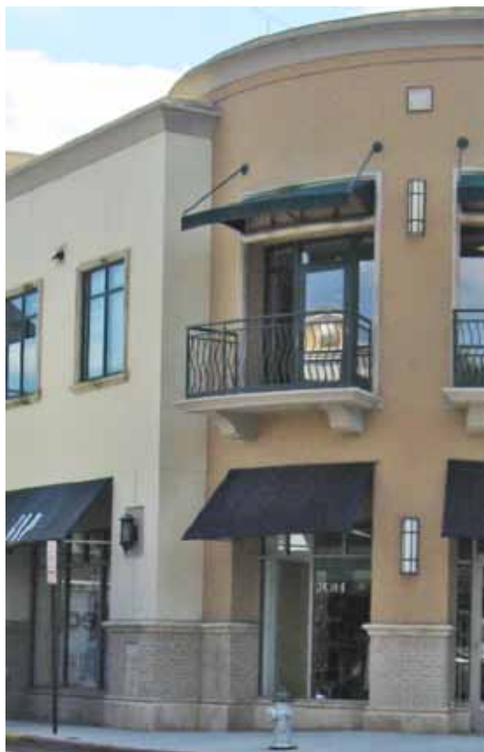
Incorporate a base, middle and cap into building design where this is established along the street wall in adjacent buildings.
