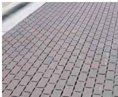
Use permeable materials for portions of a surface parking lot in order to reduce on-site run-off.
