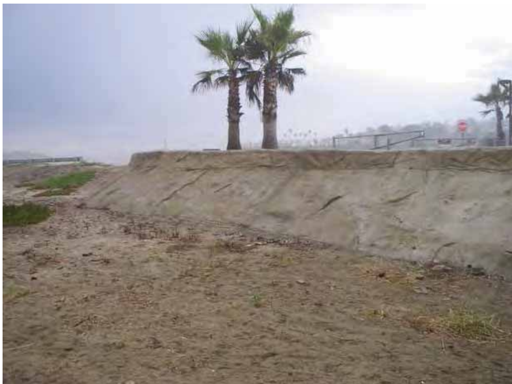
Figure 2-7 Example of Naturalized Bedrock Faux Finish on a Coastal Structure
