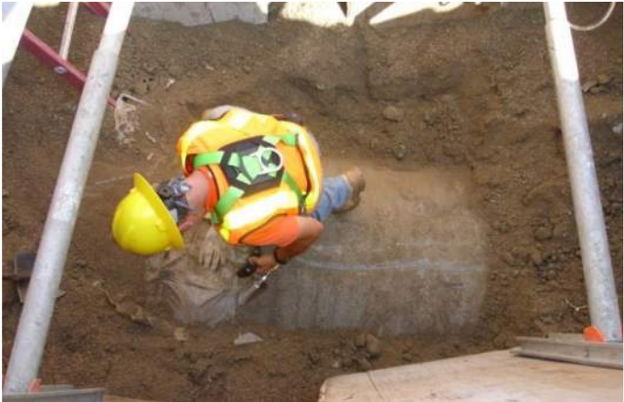
Figure 3. Example of Targeted Excavation and Measurement of Pipe Wall Thickness
